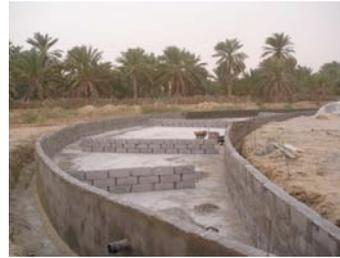
Figure 7c. Buffer walls to ensure sewage water's proper residence time and avoid short-circuiting.
